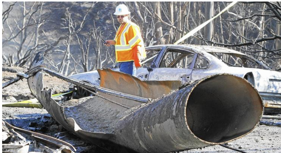
20 “The morning after the 2010 explosion in San Bruno, 21 a PG&E utility inspector looks at the gas main that ruptured. (Don Bartletti / Los Angeles Times)”
