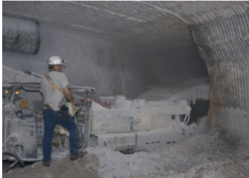
An underground chamber at the WIPP facility.
