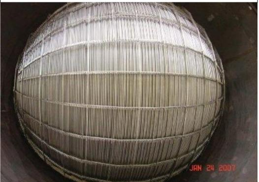
54. In order to make room for the 377 tubes, Edison removed the egg crate tube support and stay cylinder parts of the steam generators stabilization system:
